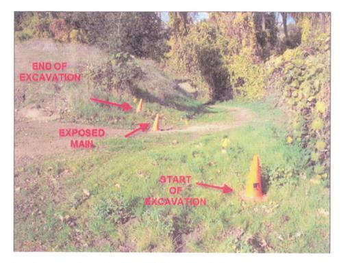
1. Photo showing the exposed gas pipeline and the extent of the excavation that will be required to lower the gas pipeline 36" below the grade.
